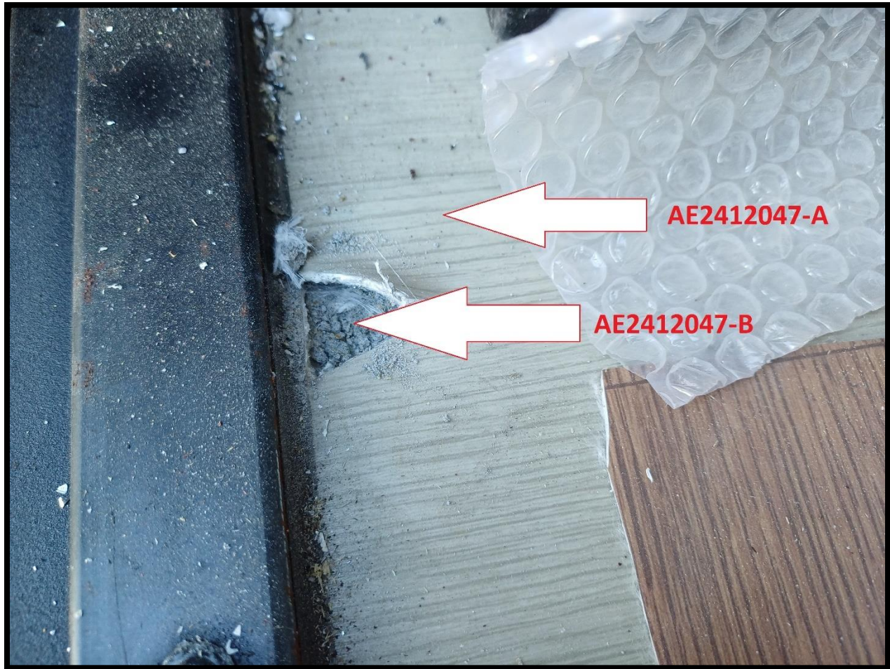
Figure 2: Vinyl floor covering/fibro cement sheet
